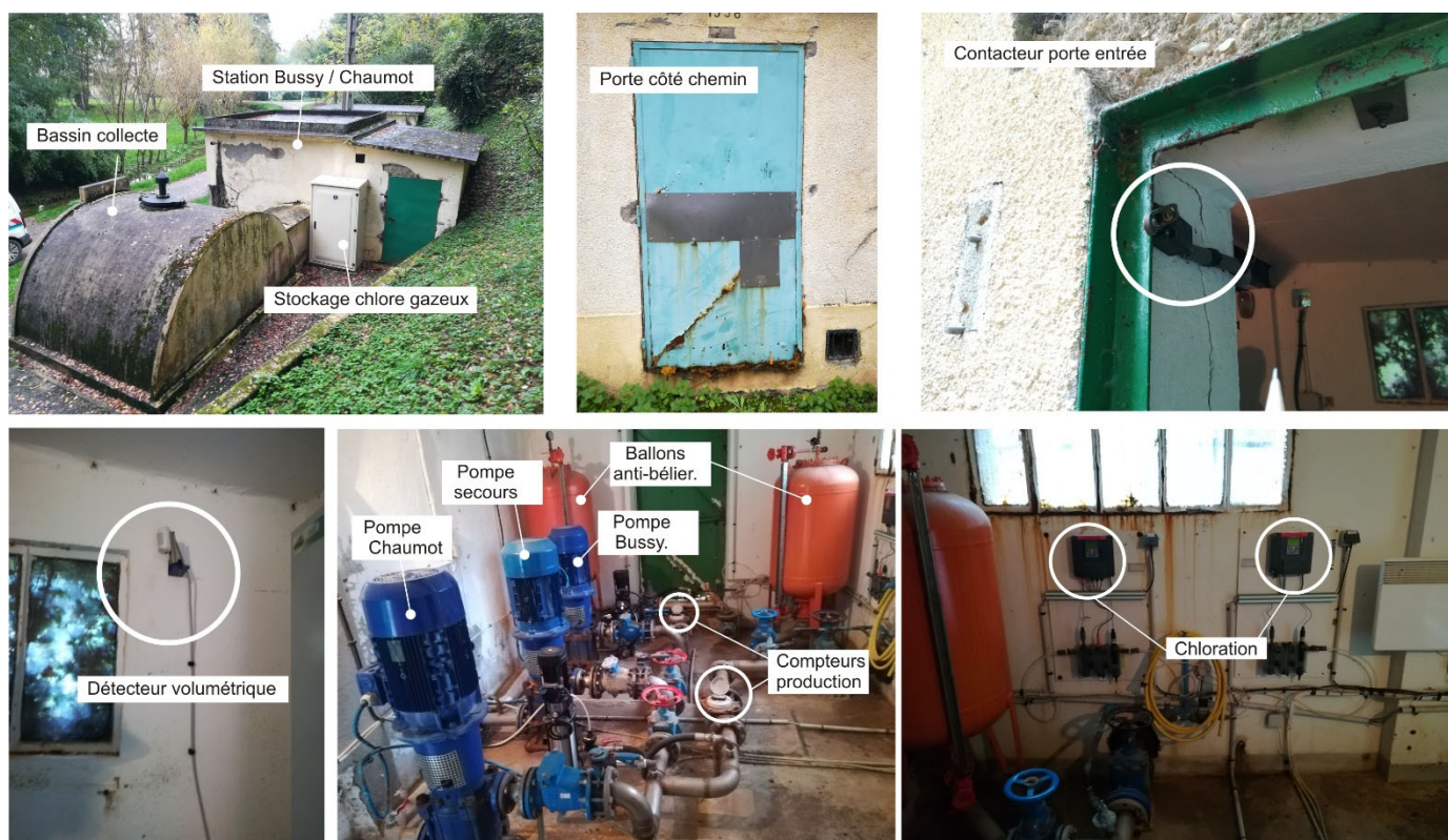
Figure 15 : station de pompage de Bussy-le-Repos / Chaumont.
